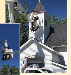
The louvres for the bell tower have been rebuilt and replaced. It's been a long process removing the old wooden louvres, making new metal ones, and re-installing them. A big thank you to Ricker Olson and Phil White for the many hours over many months they have spent planning, measuring, constructing and not to mention finding a way to get to the top of the tower. We also want to thank Phil Ehlers and Shepherd Fire, Buckley Reynolds, and Travis Dennison for their time and equipment.
